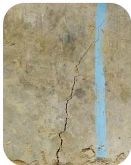
Crack pattern in unreinforced earth block
