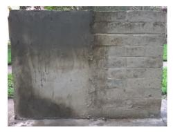
Masonry wall after application of soil-cement mortar and cement paste
