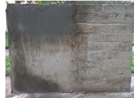
*Masonry wall after application of soil-cement mortar*
